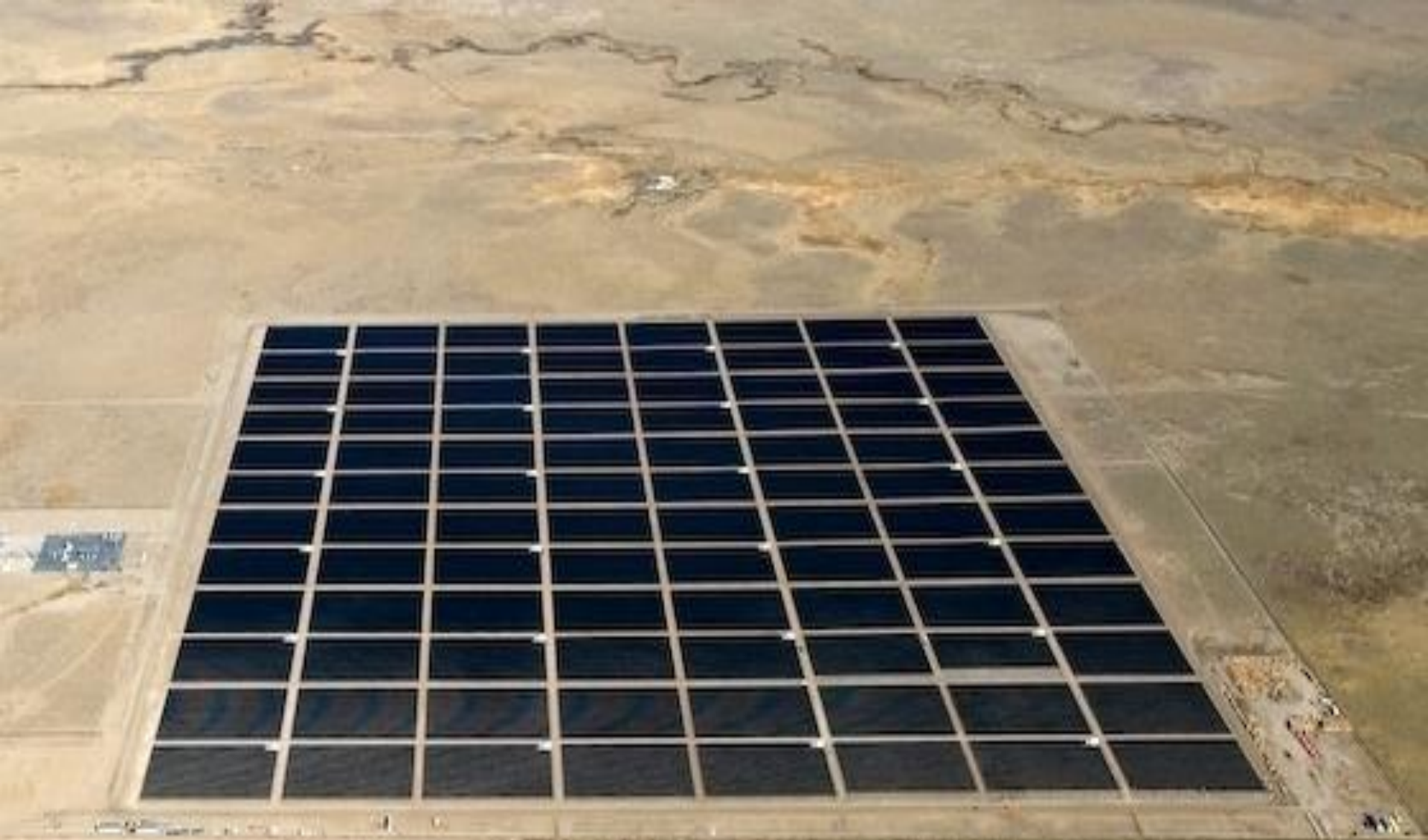
Tri-State G&T Cimarron Solar Project (30 MW)
