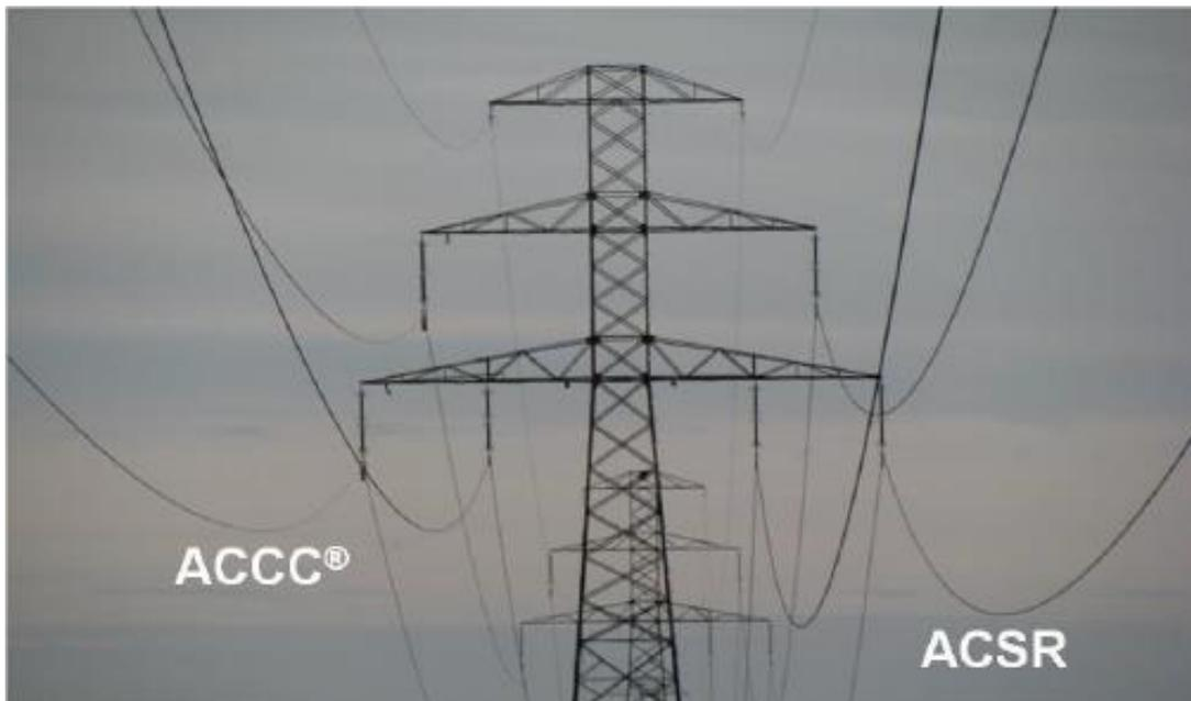
CTC Global, for example, developed an ACCC cable that has 28% more aluminum compared to an ACSR cable of the same size, which allows the cable to carry more current while suffering lower power losses [4]. The image below shows a CTC ACCC cable compared to a traditional ACSR cable of same size.
